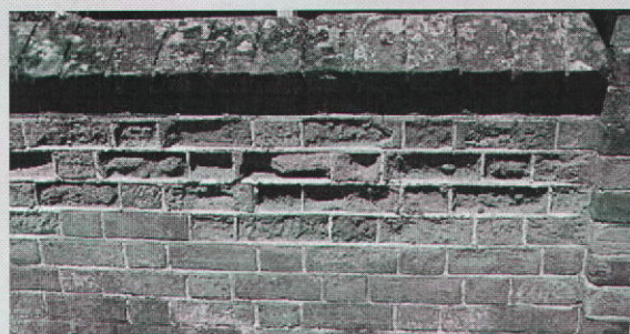
Image: An extreme case of brickwork fretting.
