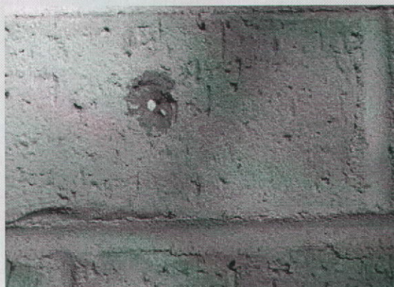
Image: An example of a large lime pit on brickwork.
